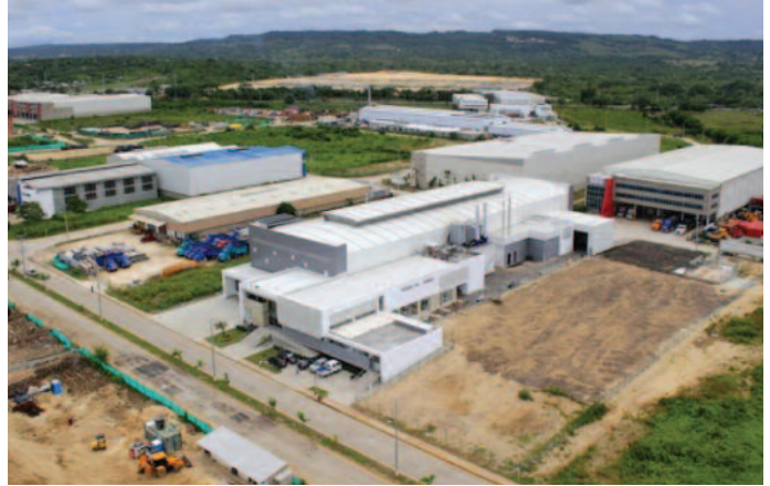
Marathon's 40,000 sq. ft. manufacturing facility opened in 2014 and offers the ability to double capacity
